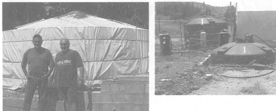
Fig. 4.10. (A) The author Gad Degani (left) and a colleague standing outside the greenhouse where the water supply filters and tanks are located. (B) Containers for storing water before use in fish tanks (1) and carbon filter (2) for removing poisons, especially chlorides.
